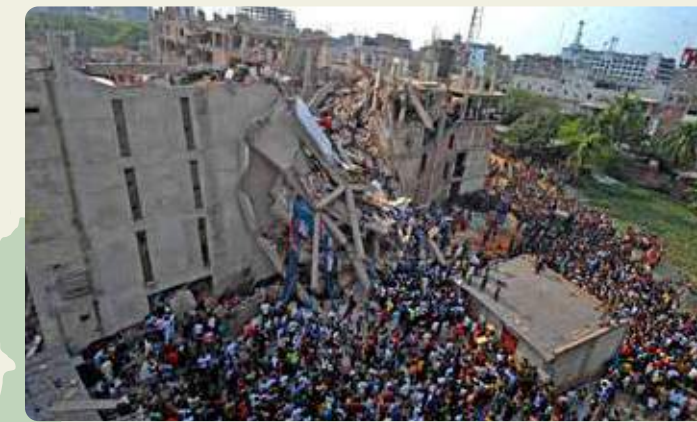
Factory collapse in Bangladesh kills 1,100 workers
